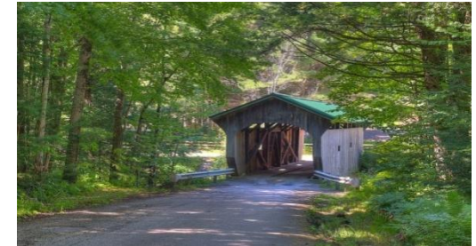
Morgan Covered Bridge, Belvedere, VT
